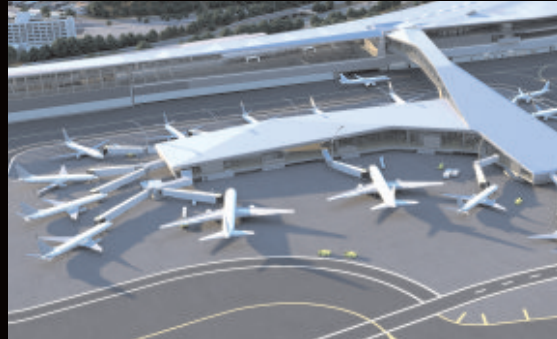
NAVI MUMBAI INTERNATIONAL AIRPORT
